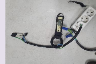
After installing ENSPD (2mA)
