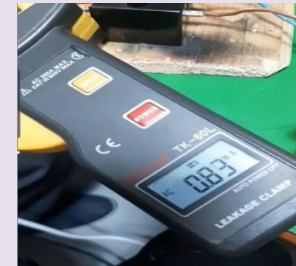
After installing ECSPD (0.83mA)
